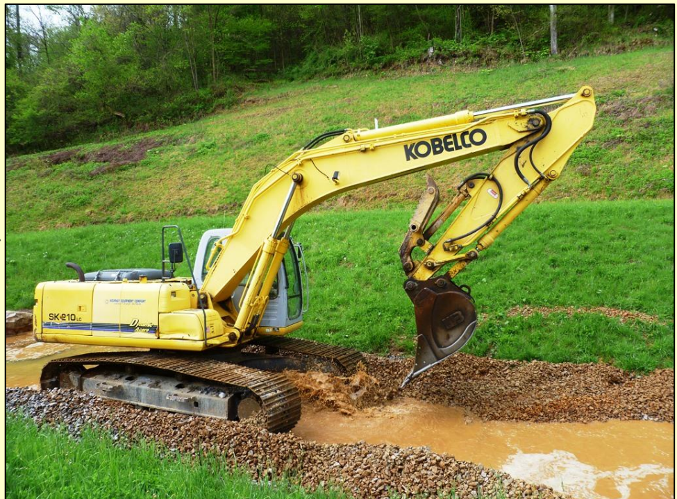
Art Grguric, BCWA Wetlands Coordinator, “fluffs” limestone at Big Run #8 to remove armored iron and improve the system’s function.
